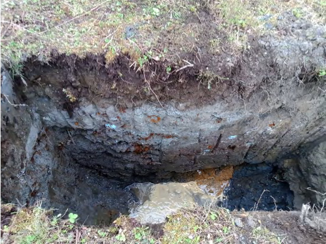
Photograph 5: Excavation at TP12.
