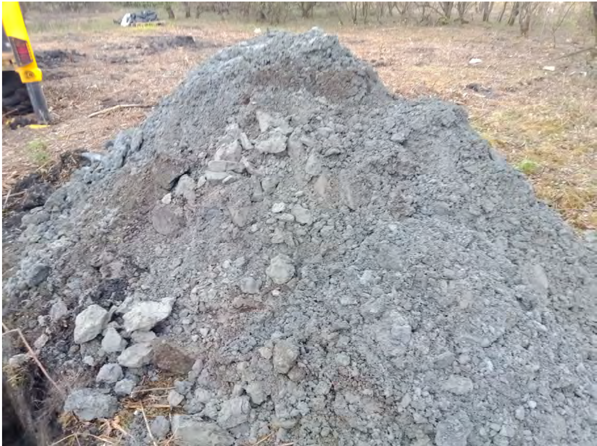
Photograph 6: Excavated materials from TP13.
