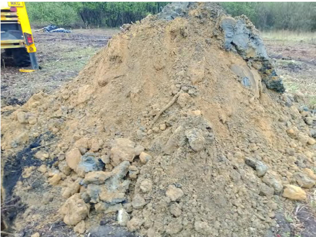
Photograph 2: Excavated materials from TP03.
