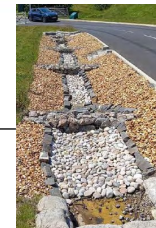
Gravel-based swale / trapezoidal ditch
