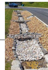
Gravel-based swale / trapezoidal ditch
