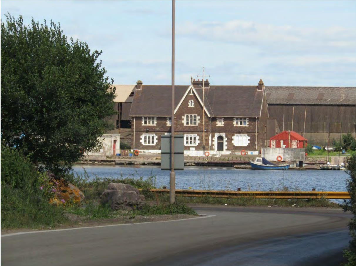
Image EDP A1.1: View north-west of the Grade II listed Harbour House, illustrating evidential and aesthetic values, as well as its visibility from the north-west boundary of site.
