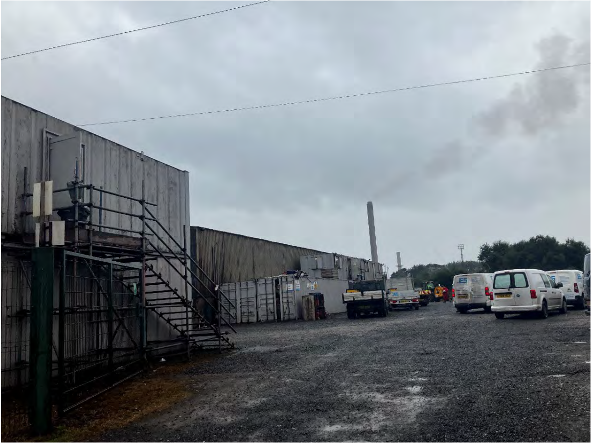
Image EDP A1.15: View west of modern, temporary buildings within the Davies Cran Hire portion of site.
