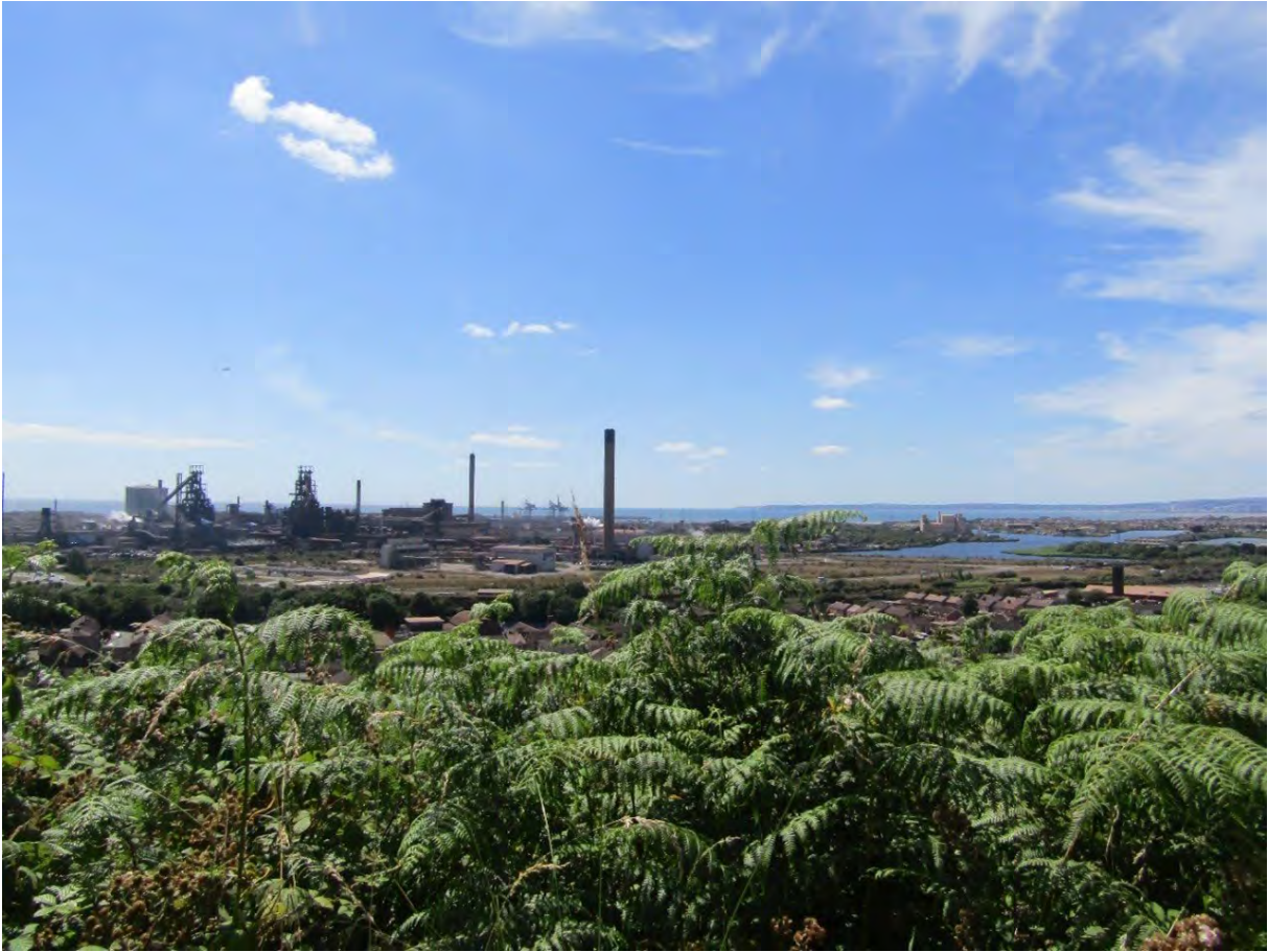
Image EDP A1.9: View west from HLCA 003, illustrating views towards the site can be achieved, but within a landscape already overwhelmingly defined by industrial form.
