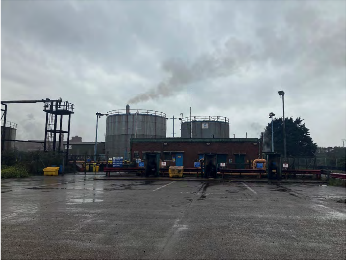
Image EDP A1.16: View north illustrating brick and cylindrical buildings within the Davies Crane Portion of site, which likely have mid to late 20 th century origins.
