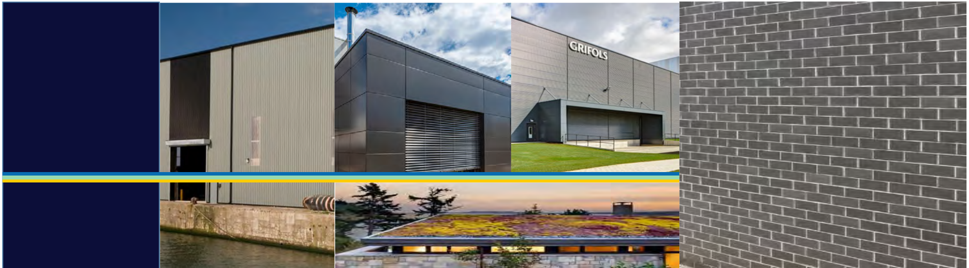
Figure 78 - Colours and Materials – For the buildings. Materials include insulated panels used chiefly on functional buildings and grey bricks used on administration buildings. Feature colours, used sparingly, and selective are based on LanzaTech corporate colours. The emphasis in colour selection is on ensuring the overall development is discrete when viewed from the wider Port Talbot area and creating low landscape and visual impact.
