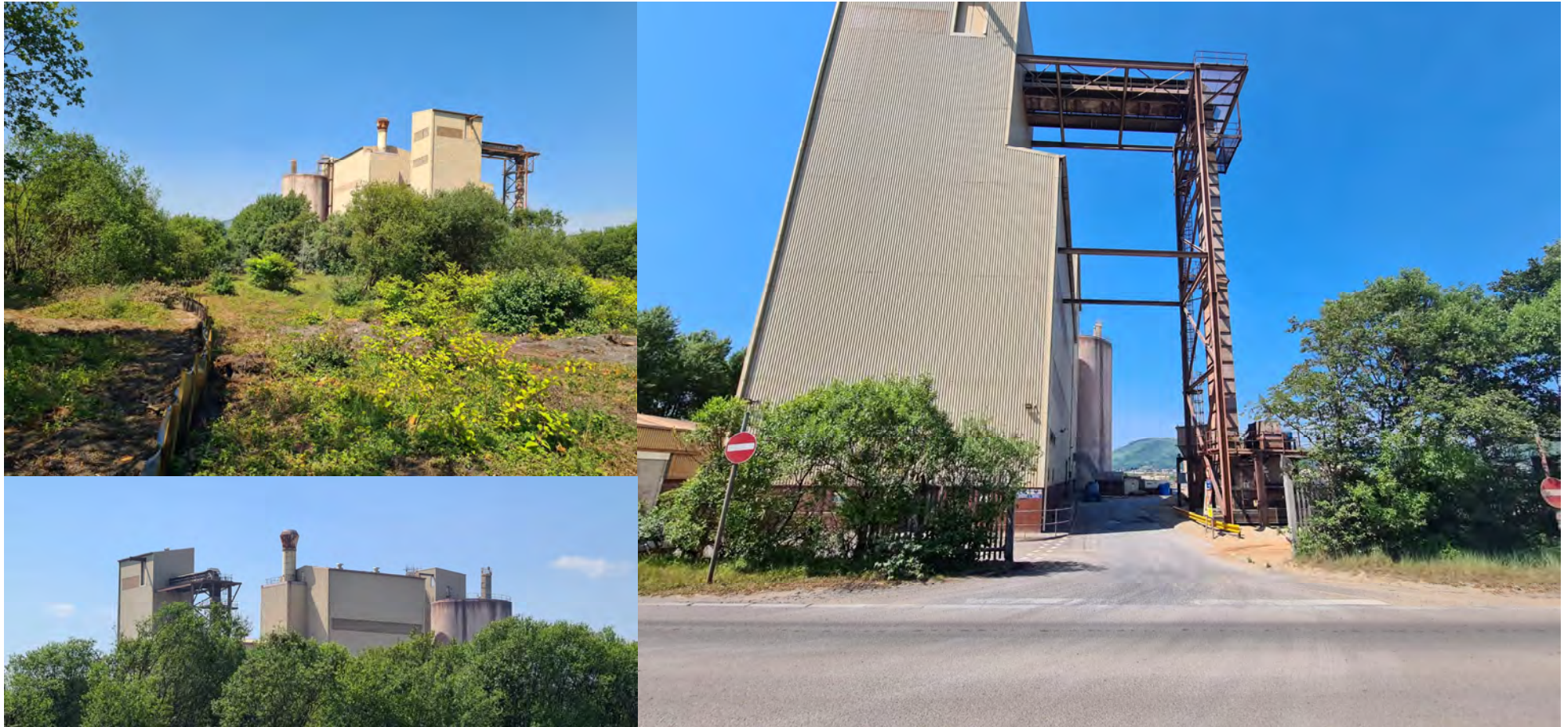
Figures 19 to 21 – The cement factory, operated by Hanson / Heidelberg.
