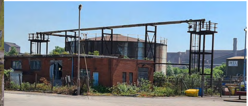
Figure 88 (Below) – Typical buildings in the area of demolition are low level, industrial use and constructed of masonry, concrete and steel.
