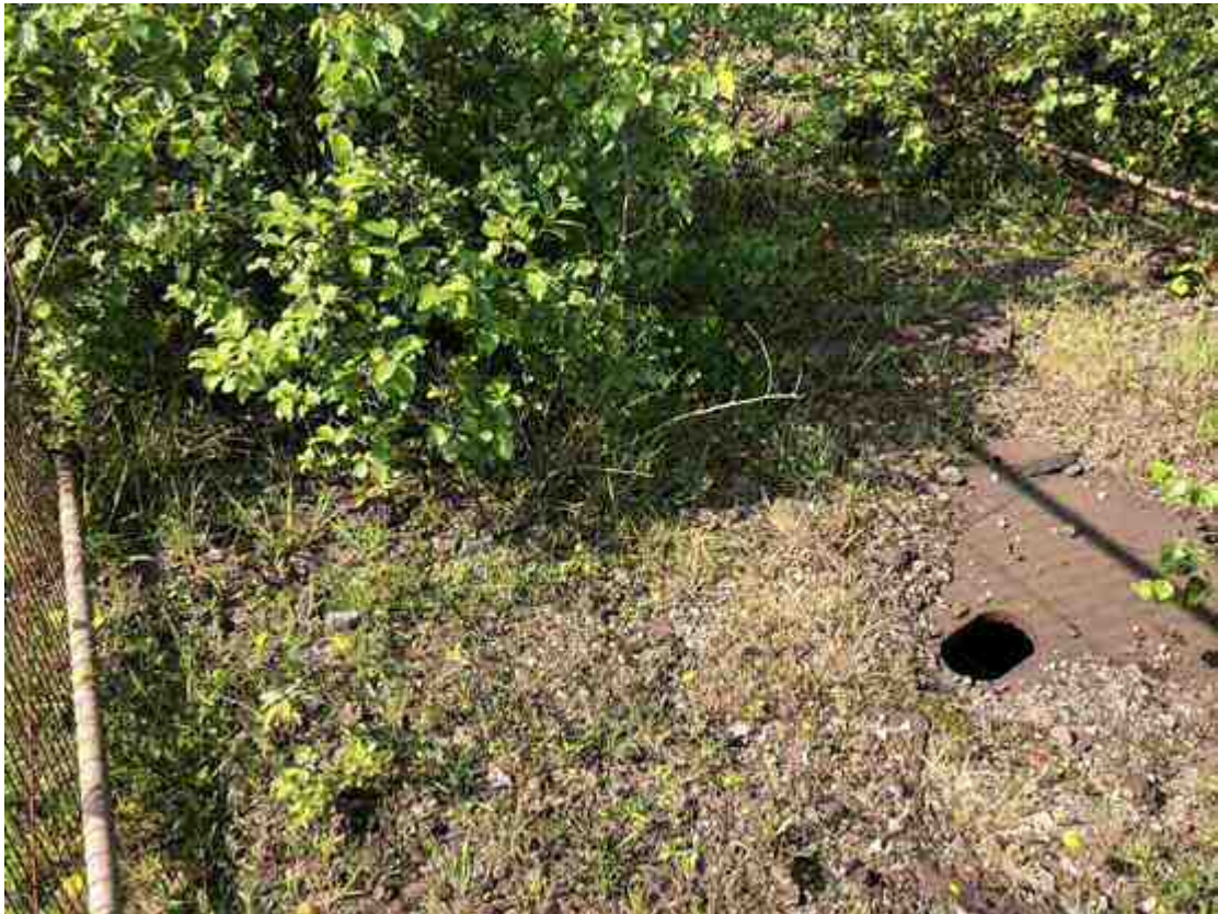
Photograph 13: View of large metal covers currently fenced off and located within the western site area.
