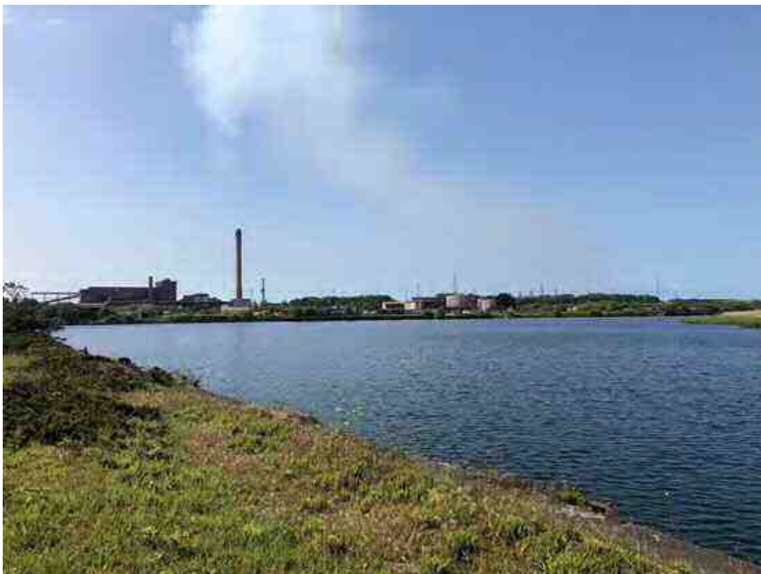
Photograph 8: View from northern site area, facing south-west across the wharf.
