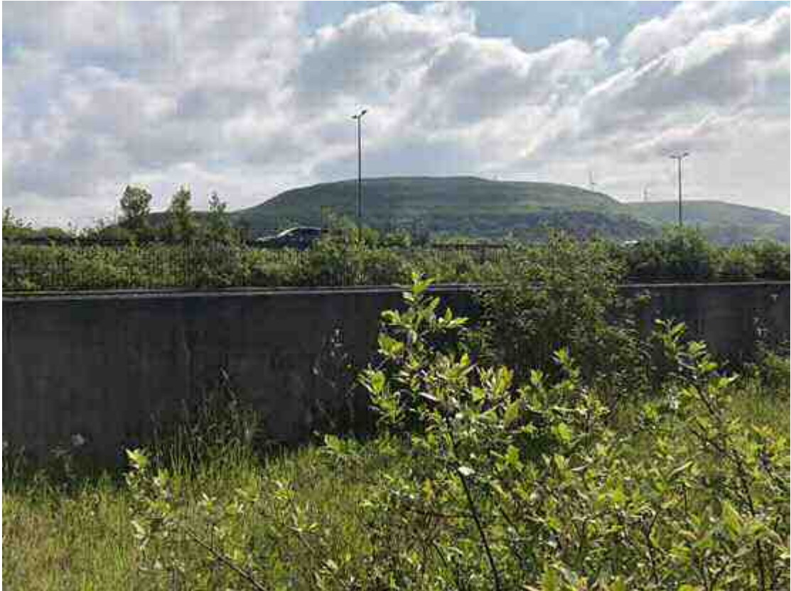
Photograph 6: Interlocking concrete blocks, located north and north-east of the site, formally used as an access road leading to the northern gate.
