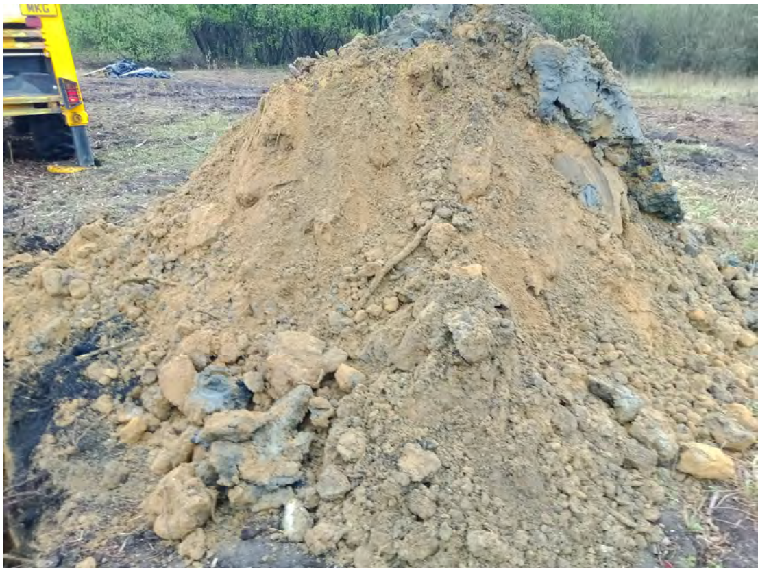
Photograph 2: Excavated materials from TP03.
