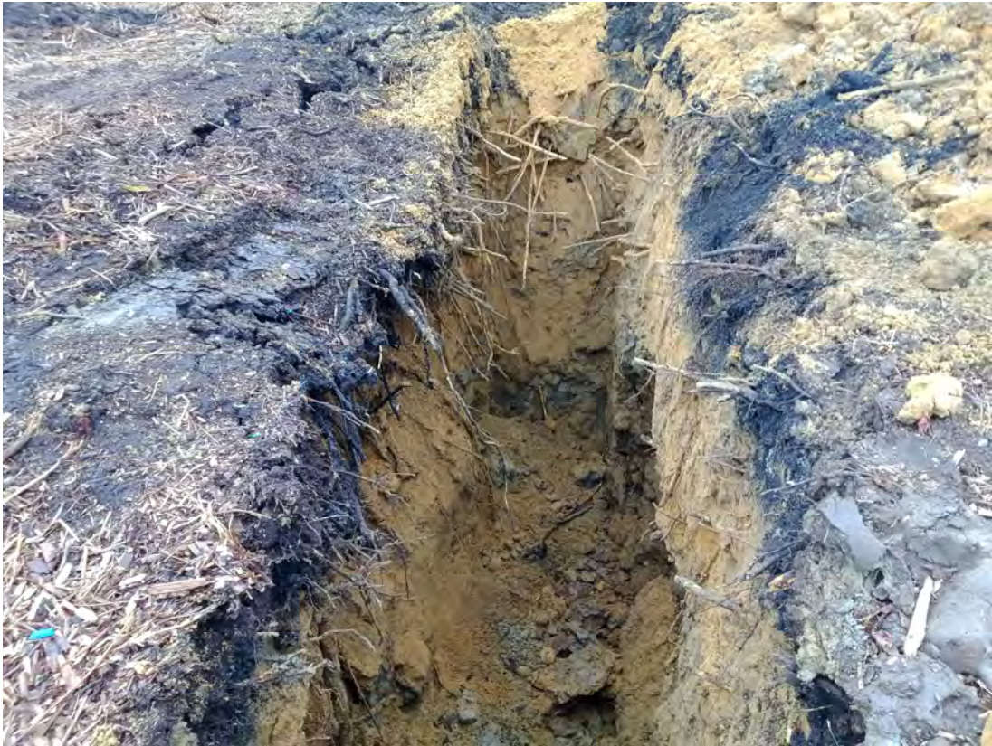
Photograph 1: Excavation at TP03.
